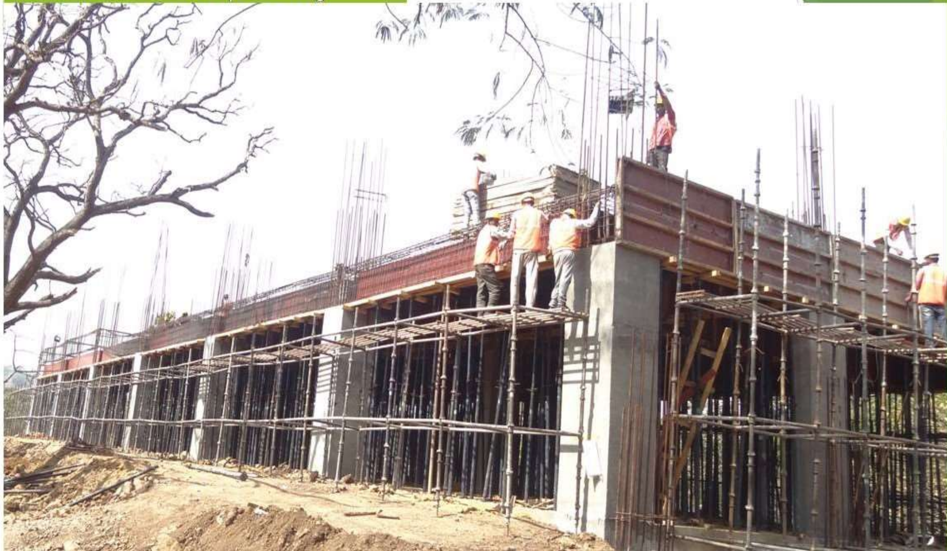
Maintenance Workshop Building -
