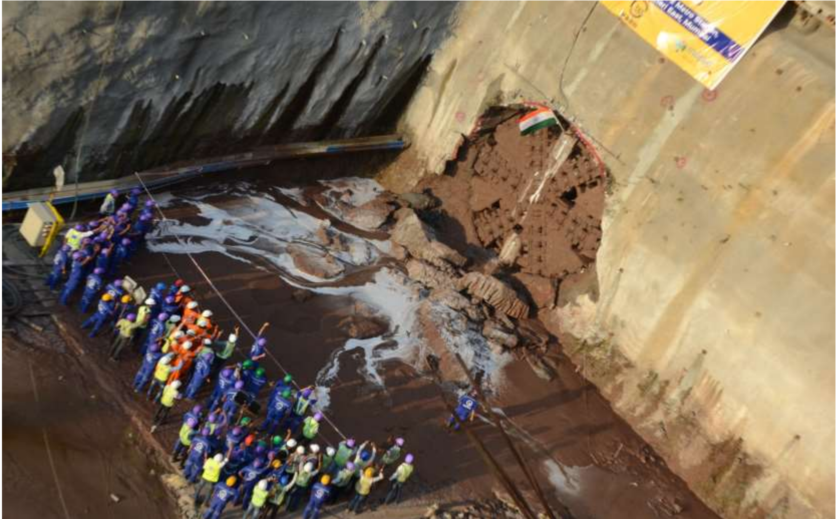
1 st Breakthrough – CSMIA-Terminal-2 station
