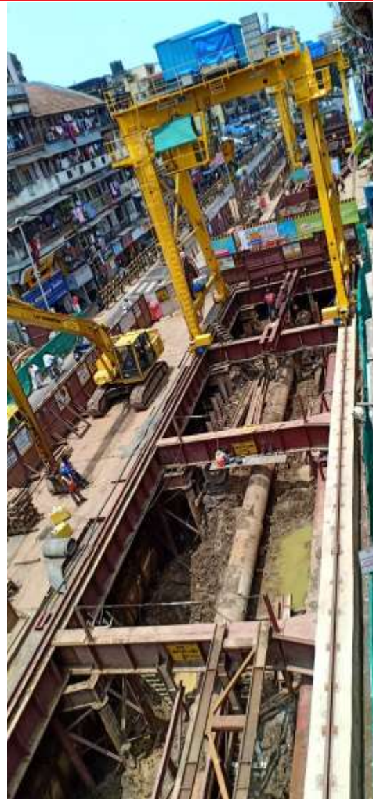
Grant Road Station
