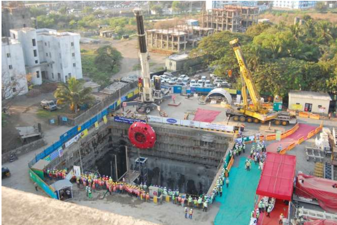
Overview of Launching Shaft site
