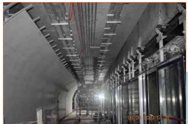
SHC MEP Conduiting work at NATM Side
