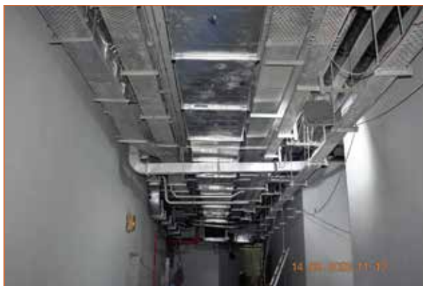
SCP Cable tray and Duct Work
