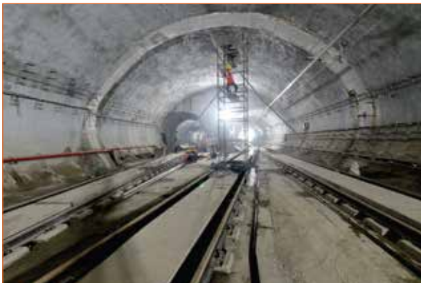
Work in progress at Sahar Crossover
