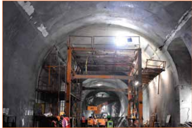
Dismantling work_SHC NATM
