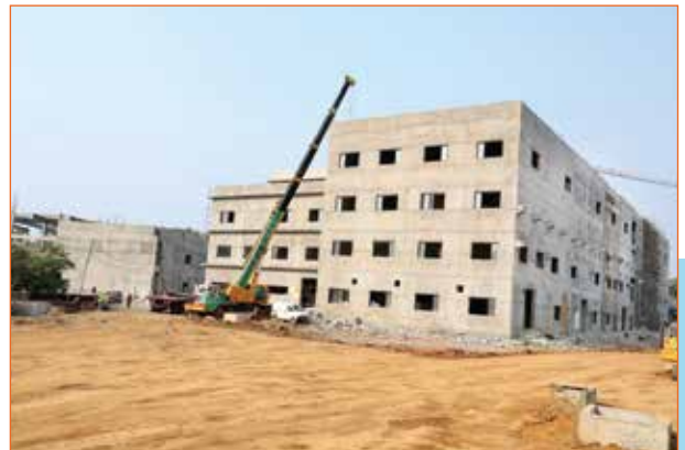
Work in progress at Aarey Car Depo
