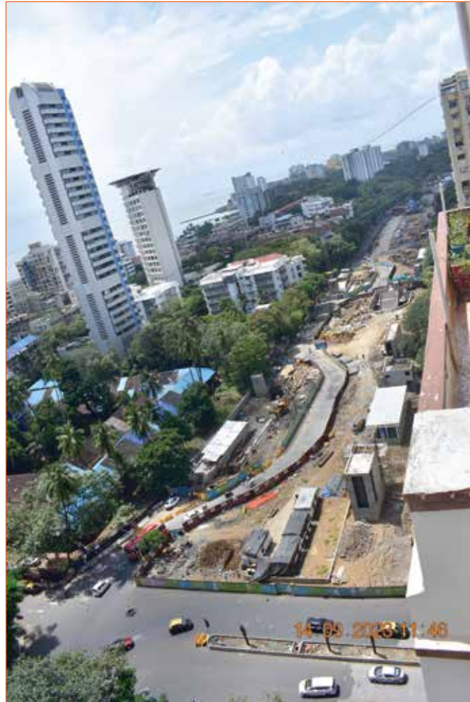
SCP Aerial View
