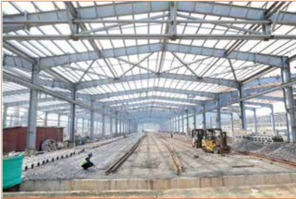
Work in progress at Aarey Car Depot
