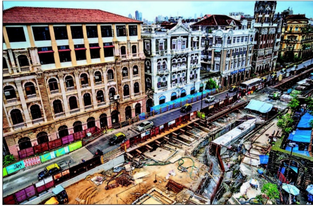
Work in progress on Metro Line 3 and Hutatma Chowk station near Flora Fountain.
