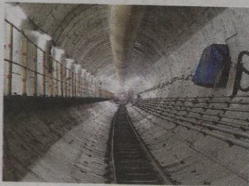
The tunnel at Metro line III
