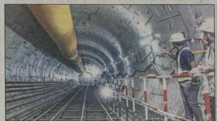
out tunnelling in grade 4 and grade 5 (broken rock geology with a water body above). The TBM machines being used here are capable of dealing with such situations. Moreover, to overcome monsoon challenges in the station area, we have installed de-watering pumps to flush out inundated water," said Gupta.
