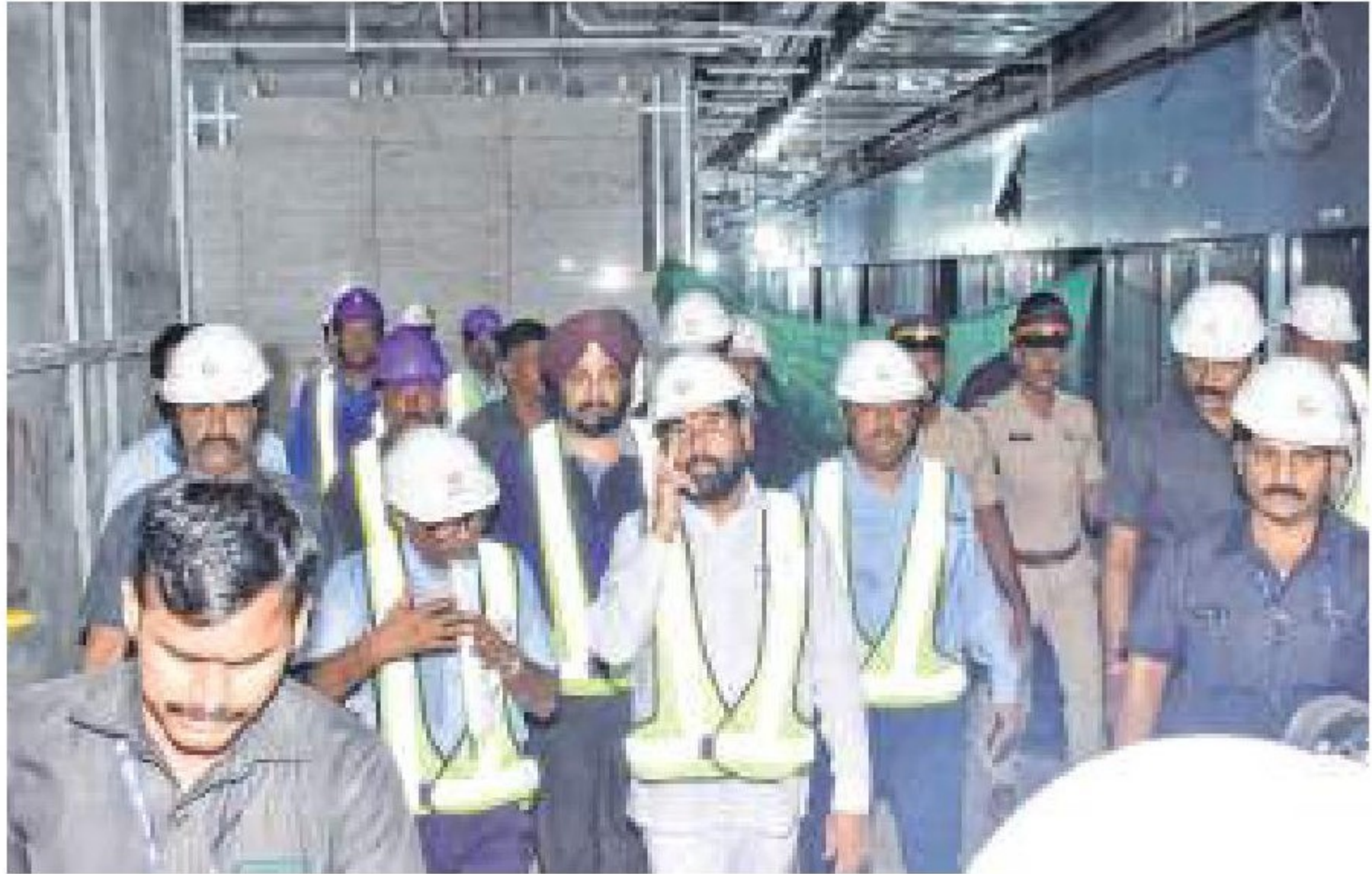
Chief Minister Eknath Shinde and other officials inspected the Metro 3 underground project at Vidhan Bhavan Station late on Tuesday night
